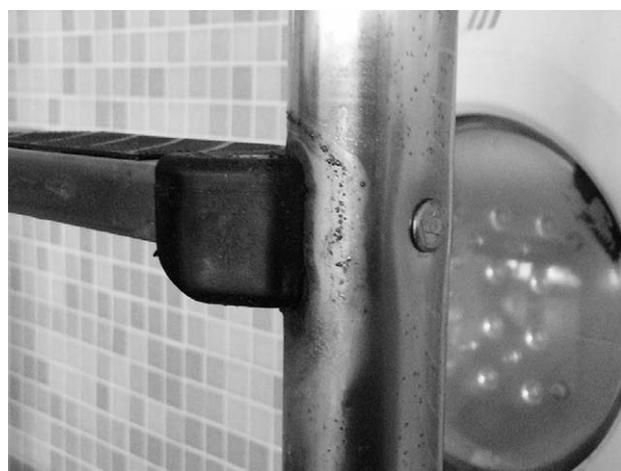
**Figure 2:** Rust on the vertical holder around the bolted-step connection
