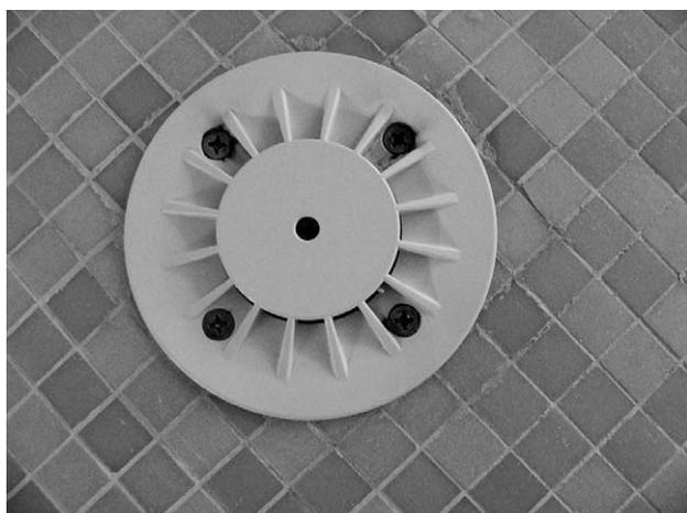
**Figure 1:** Rusted cross-head screws at the bottom of the pool
