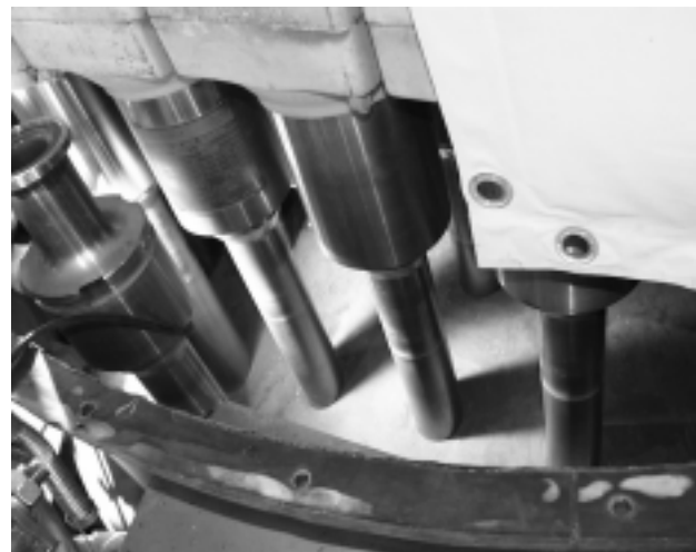
Slika 5: Površina reaktorske glave okoli kontrolnih palic št. 10, 31, 23, 18 in 22 Figure 5: Reactor surface around control rods 10, 31, 23, 18 and 22
